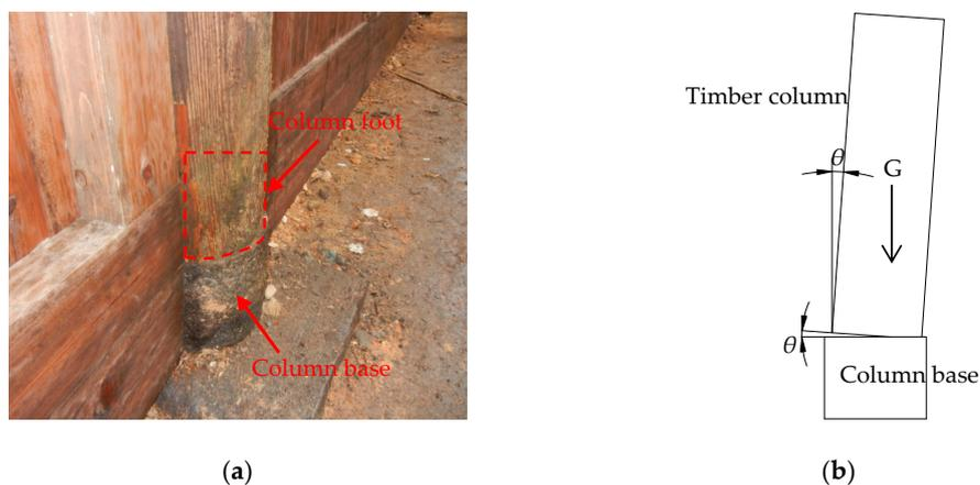
**Figure 4.** Connection type of Chinese traditional timber structure base: (a) Flat pendulum floating column foot; (b) A simplified model of tilted timber column.
