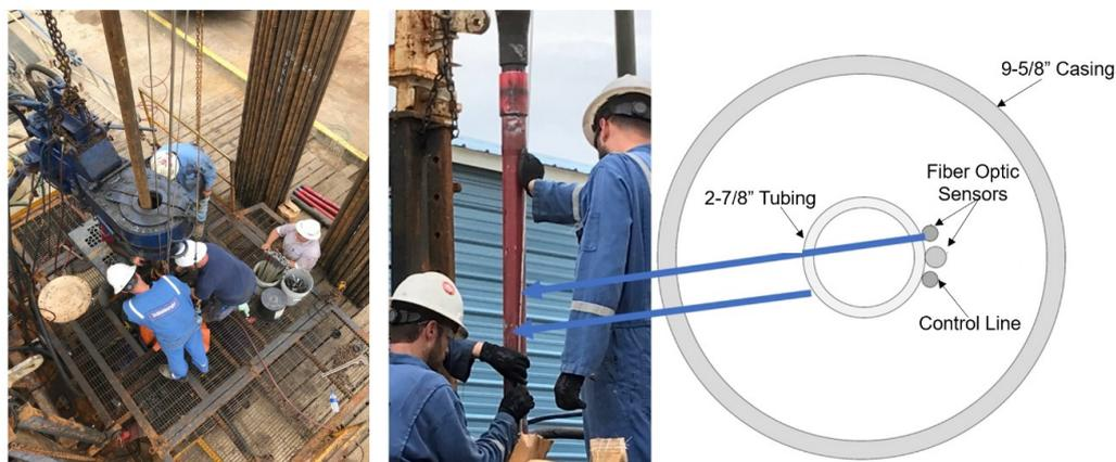
**Figure 6.** Test well workover and fiber installation performed by Schlumberger.
