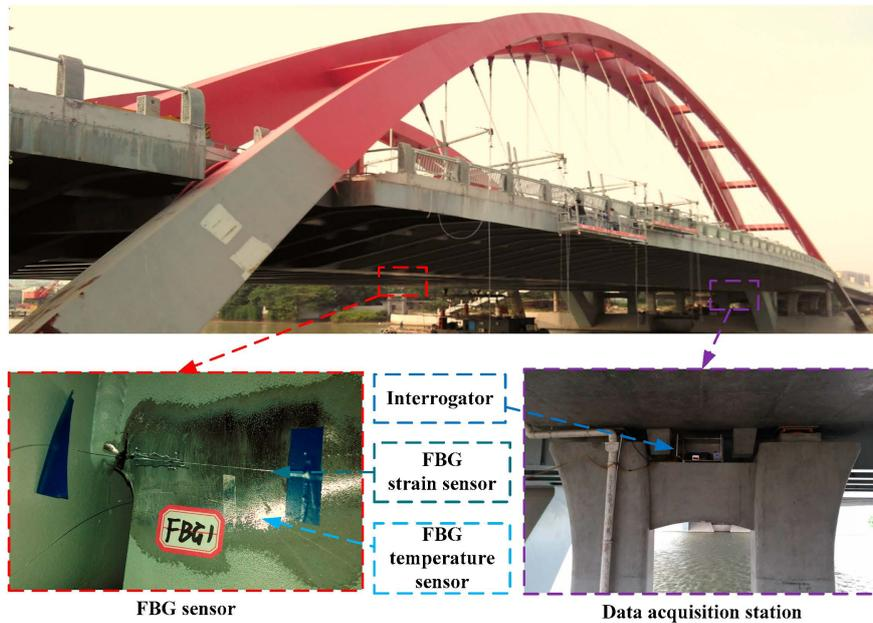
**Figure 9.** Deployment of structural health monitoring (SHM) system based on fiber Bragg grating (FBG) [151].
