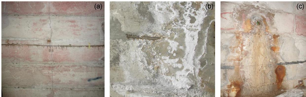
**Figure 10.** Crack on the tunnel wall crossed by the glued fiber (a); target swelling and salt precipitate accumulation (b); salt precipitate accumulation (c).
