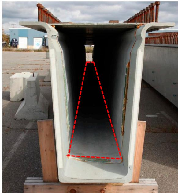
**Figure 3.** A picture of one bridge girder. The red mark indicates the location of the sensing textile.
