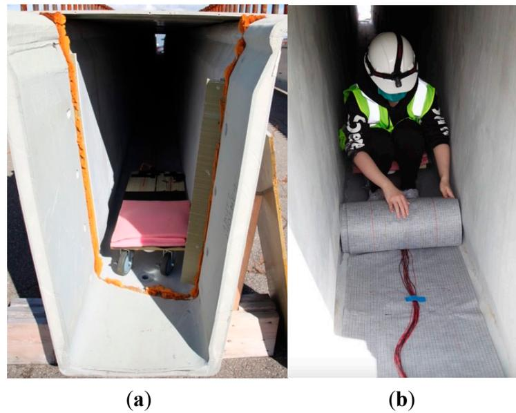
**Figure 5.** Pictures of fiber optic sensing textile installation. (a) The modified slider fits inside the girder. (b) One of our group members was unrolling the sensing textile inside the girder.
