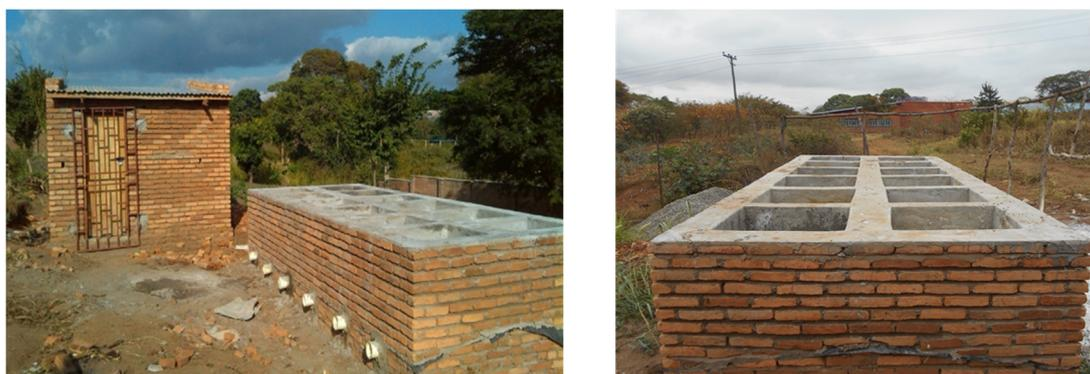
**Figure 1.** Unplanted drying beds prototype.
