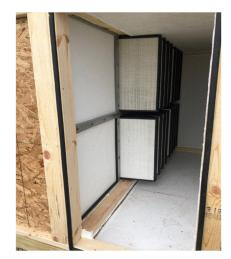
Figure A5. Picture of the inside of the MERV filtration unit.
