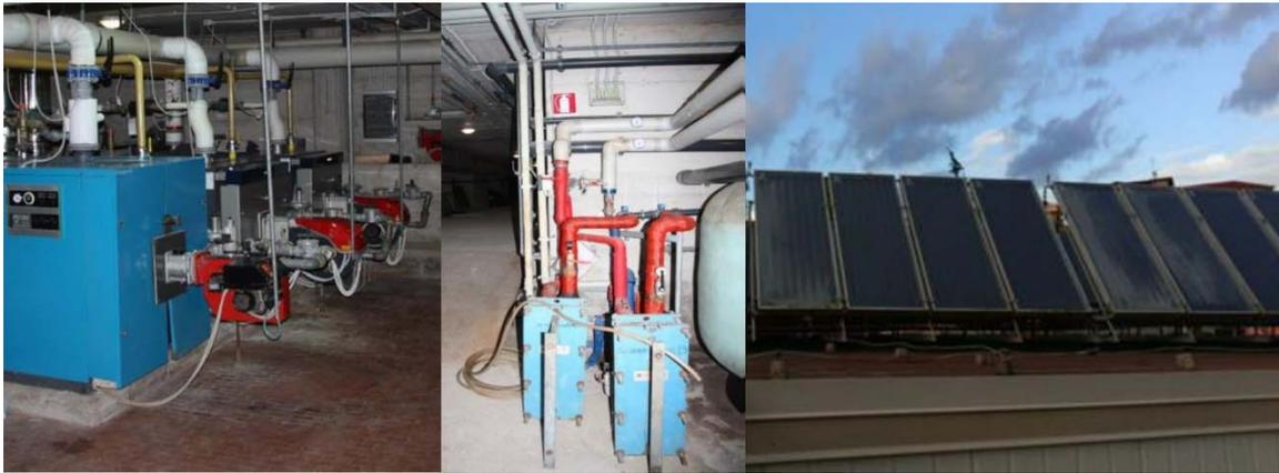
**Figure 3.** Main components of the swimming pool existing installation: natural gas boilers (**left**), swimming pool heat exchangers (**centre**), thermal solar collectors (**right**).
