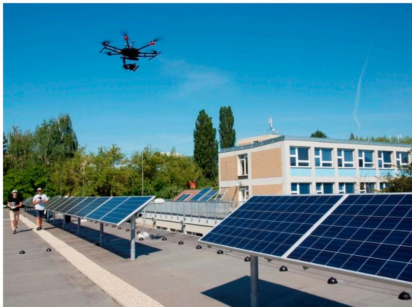
**Figure 1.** Photovoltaic (PV) power plant and drone during temperature monitoring.
