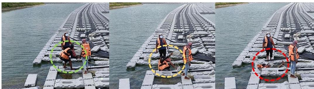
**Figure 1.** A worker is seen falling (marked in circles) due to an unstable working platform during installation of a solar photovoltaic project in India (image source: authors).
