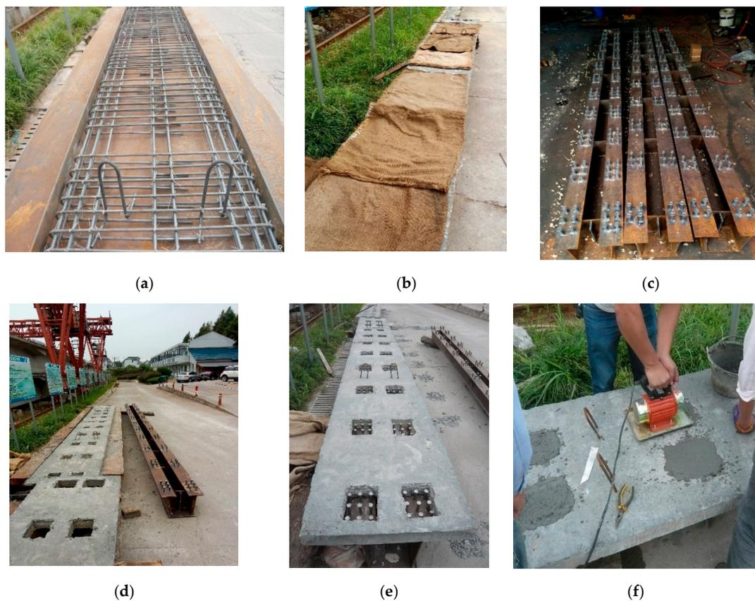
**Figure 2.** Fabrication process of the experimental beams: (a) formwork erection and reinforcing case binding; (b) casting and curing of concrete slab; (c) stud welding of test specimens; (d) completion of the concrete slab and steel U-type girder; (e) placing of concrete slab on steel box girder to make it composite; (f) reserve hole filling.
