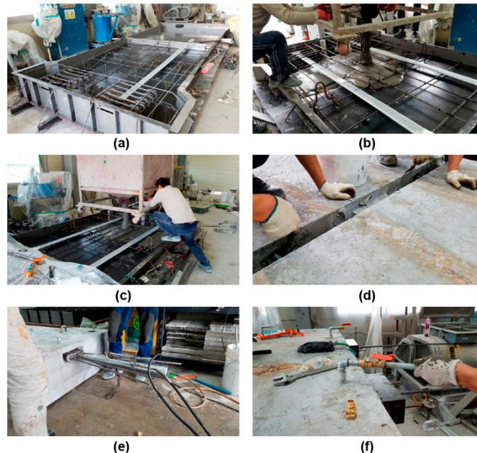
**Figure 2.** Fabrication of the specimens: (a) assembly of mold and reinforcement placing, (b) concrete casting (one side), (c) concrete casting (other side, match casting), (d) epoxy spreading, (e) jacking, and (f) grouting.
