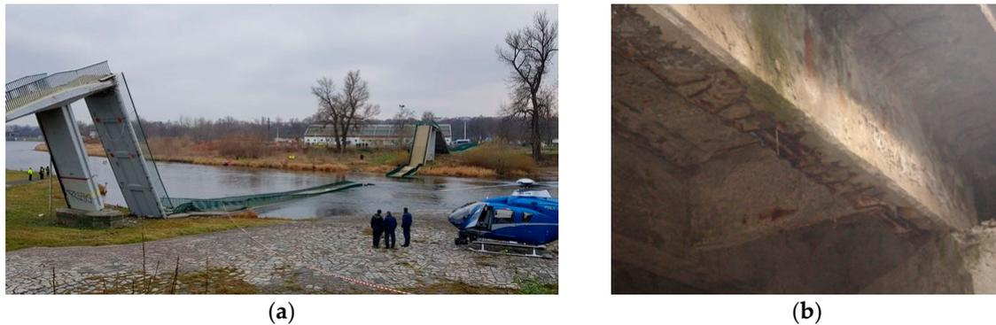
**Figure 1.** Failures of bridges: (a) collapse of the pedestrian bridge due to corrosion of prestressing cables in city Prague, the Czech Republic [3]; (b) corrosion of reinforced concrete (RC) T-beam bridge in Kolarovice, Slovakia (2006).
