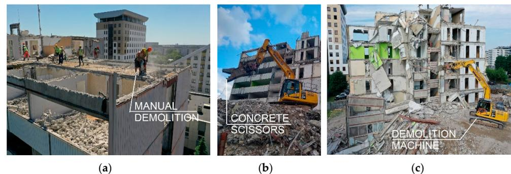
**Figure 2.** Demolition of the building: (a) manual demolition; and (b,c) mechanical demolition.
