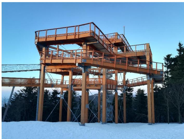
**Figure 1.** Example of a timber structure with bolted connections.
