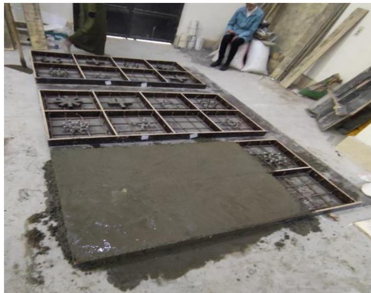
Figure 4. Wood formwork and casting work.
