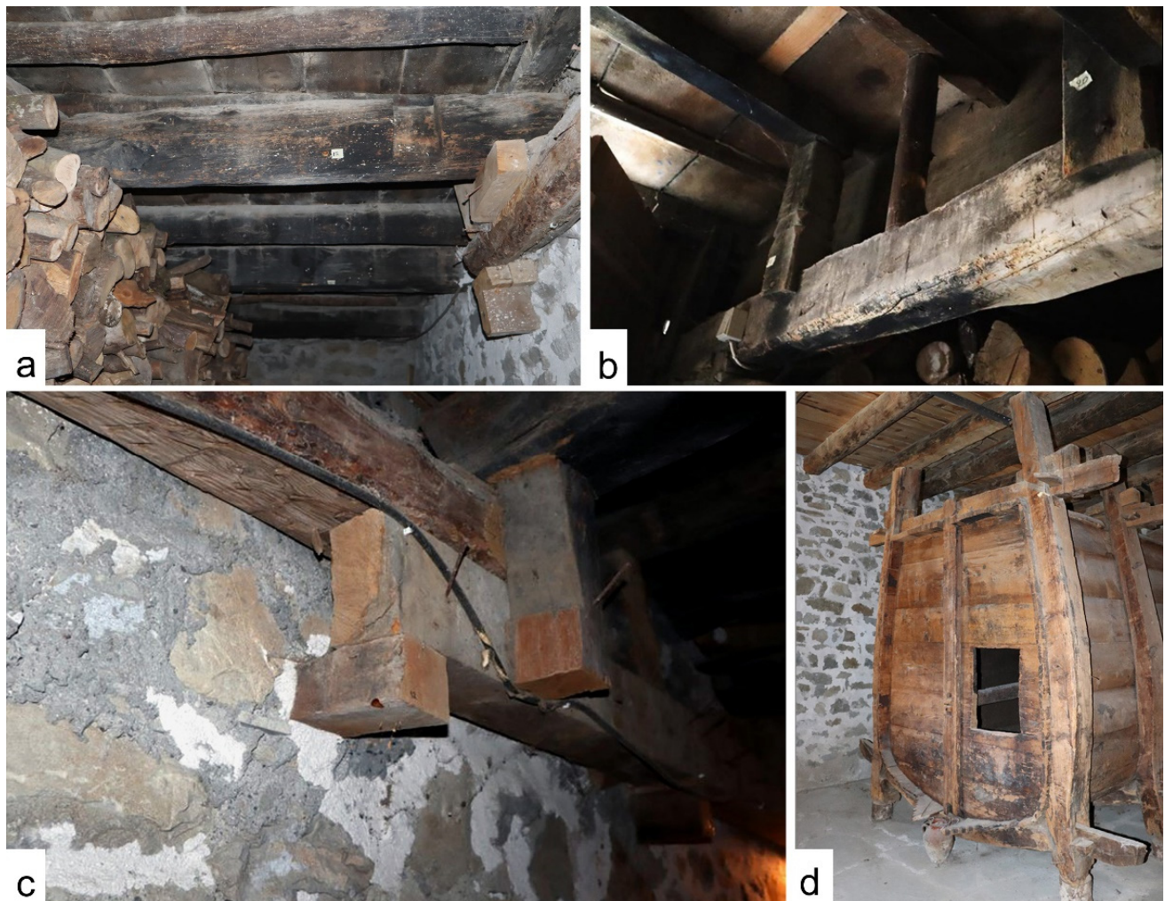
Figure 3. (a) Floor beams next to firewood, at the corridor driving to the basement in the auxiliary building; (b) vertical elements supporting the floor beams on the horizontal beam placed at the lower level; (c) cantilever beams at the lower level, supporting the floor beams with extra timbers (d) old wine barrel stored at the basement of the auxiliary building.
