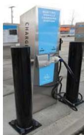
Figure 1: EVSE with Protection Barriers
