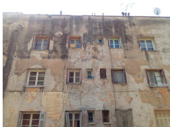
Figure 4. Deterioration of historic plaster.
