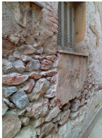
Figure 11. Morphology of the stone masonries.
