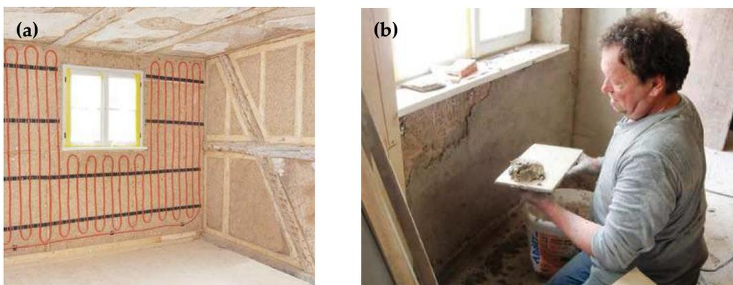
**Figure 8.** (a) Covered surface and screwing of the heating system, picture: Fritsch Knodt Klug (b) clay plastering on internal insulation, picture: Alexandra Fritsch.
