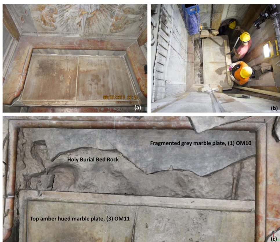
Figure 6. Description of sampling areas of marble samples (1) OM10 and (3) OM11: (a) the Holy Tomb with the top amber hued marble plate, that it is worshiped today, in place; (b) View of the Holy Tomb during the shifting out of position of the top amber hued marble plate on October 26, 2016; (c) The open Holy Tomb where it was visible: the Holy Burial Bed Rock; the fragmented gray marble plate (sampling area of (1) OM10); the, shifted out of position, top amber hued marble plate (sampling area of (3) OM11).
