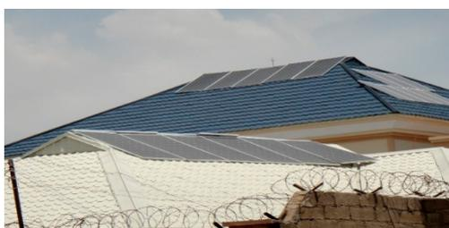
**Figure 5.** Solar PV panels mounted over a hip roof.
