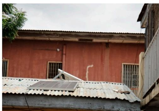
**Figure 6.** Solar panels mounted on the roof top of a bungalow house with a duplex house blocking the early morning sunrays from the east.
