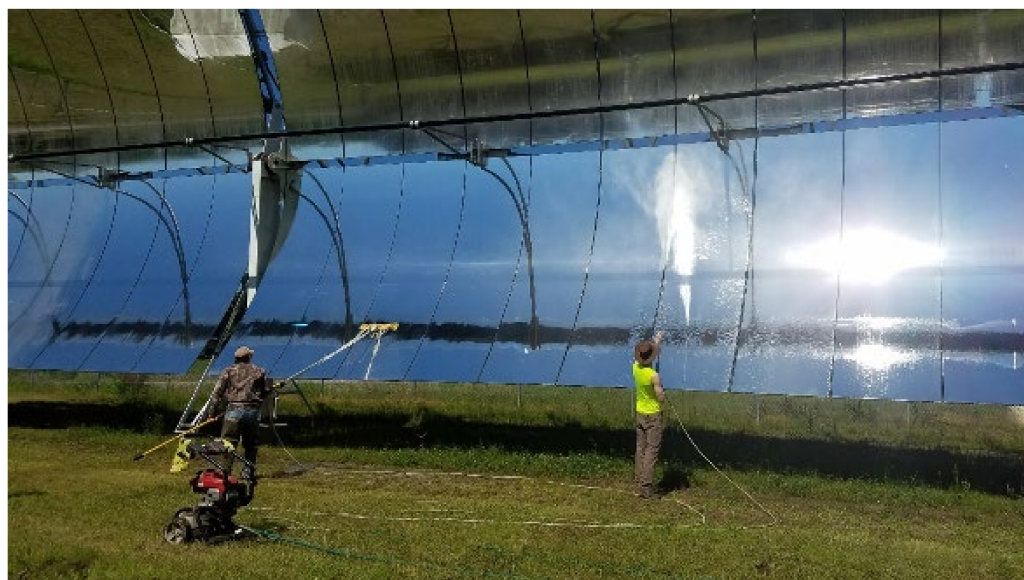
Figure 2. Solar reflector cleaning in Crowley, LA.
