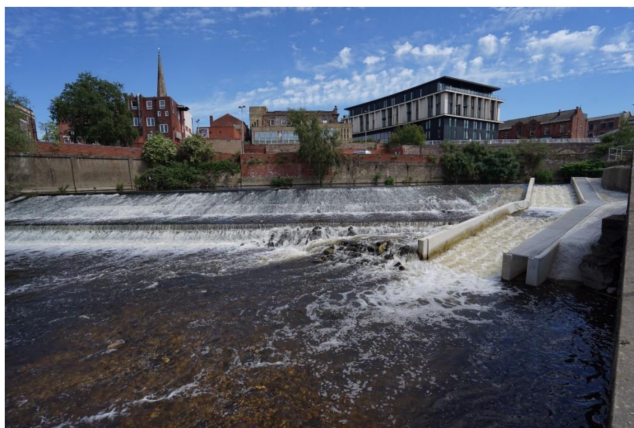
Figure 15. A Larinier fish pass built 2020 on Masbrough Weir in the River Don at Rotherham. Photograph: DCRT 2020.
