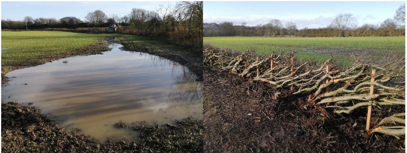
Figure 16. Examples of Natural Flood Management interventions created upstream of Chesterfield. Left: scrapes dug to intercept and store runoff. Right: Hedgerow restored to slow down the flow of runoff. Photograph: DCRT 2020.
