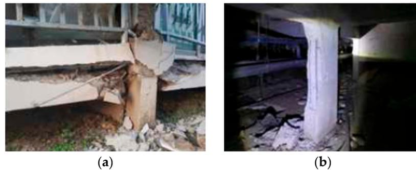
**Figure 1.** Separated joint, impact fracture, joint fracture, and short column fracture in the Dae-seong apartment complex. (a) Separated joint, impact fracture; (b) Short column fracture on the basement floor.
