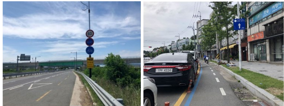
Figure 3. T2-cycle track: with a signage on the side of the road (left), T2-cycle track: tubular markers broken by parked cars (right) (Source: authors).
