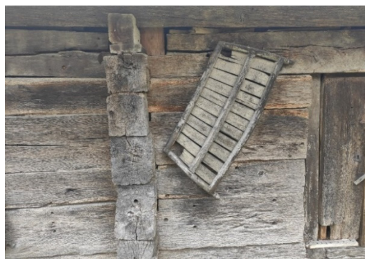
Figure 9. Facade detail showing the traditional “Croatian” joint and the still functional wooden tool for collecting and disposing of food in the village of Donja Kupčina.
