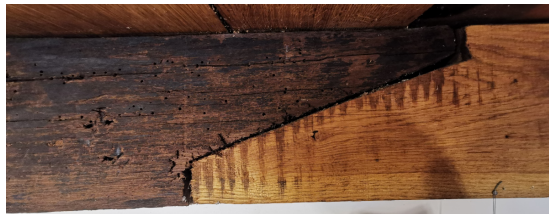
Figure 3. Longitudinal joining of wooden planks. Found in the villages of Čigoč and Krapje. Reprinted with permission from Ref. [5]. 2021 Robert Roginić.
