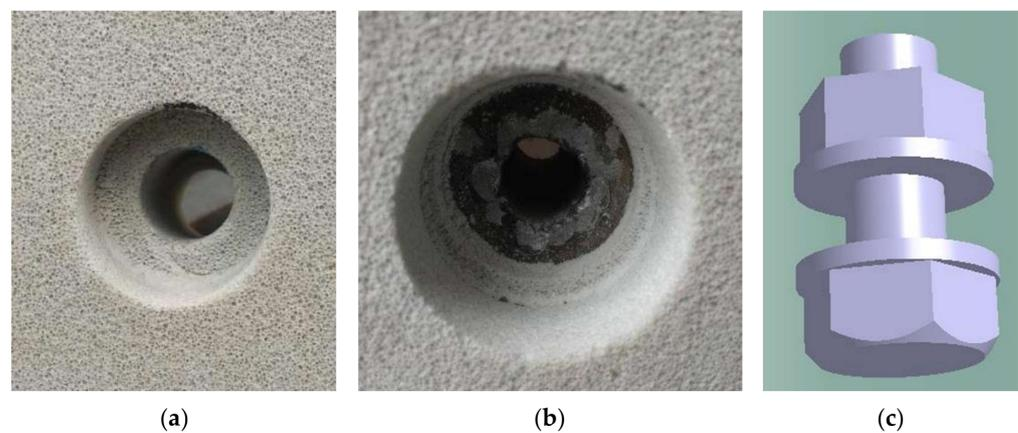
**Figure 7.** Connection structure of composite wallboard with foamed ceramic and foamed concrete: (a) penetrating round hole; (b) sleeve placed in long hole; (c) connecting bolt locking sleeve.
