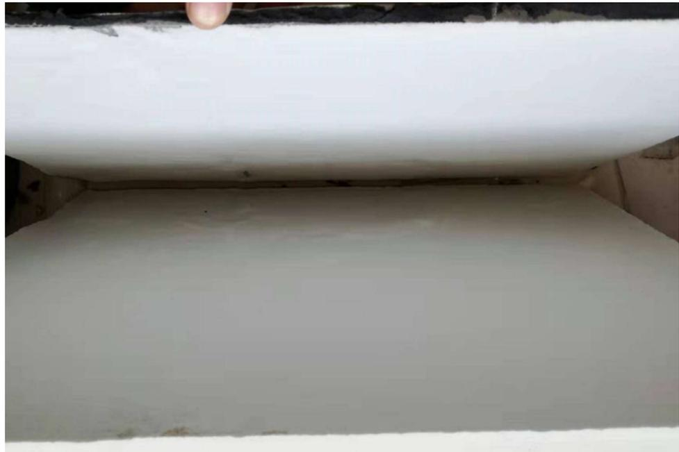
**Figure 3.** Foamed ceramic board is torn by shrinkage stress of bonding mortar.
