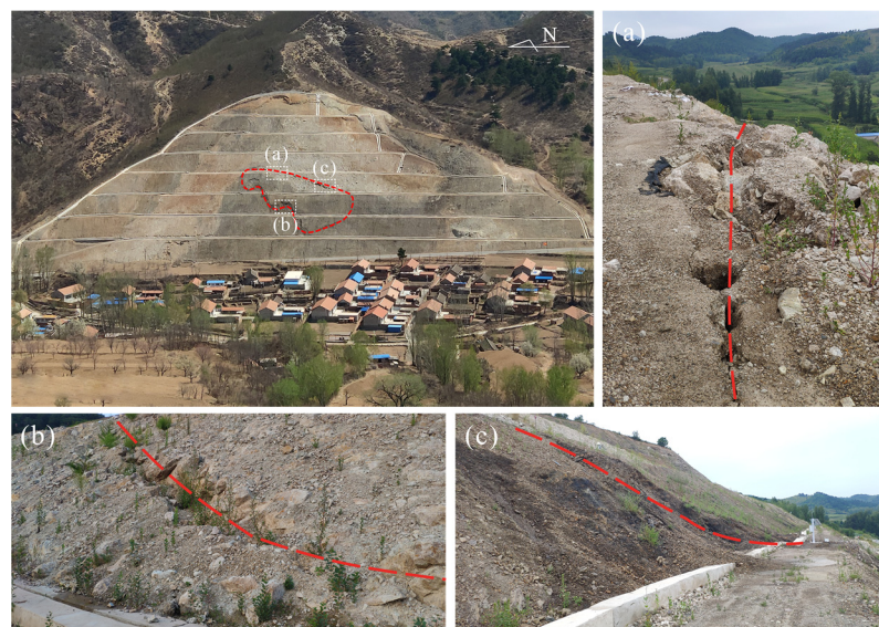
Figure 16. A secondary sliding zone developed within the Nandongzi toppling showing the connection of the (a) steep tension fractures at the rear edge of the secondary sliding zone, (b) shear fissures along the bottom sliding surface and (c) lateral scarps.
