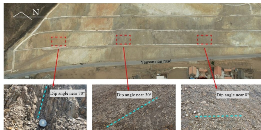
Figure 6. The deflection angle of the rock layer exposed on the slope surface, i.e., the evidence for the toppling.
