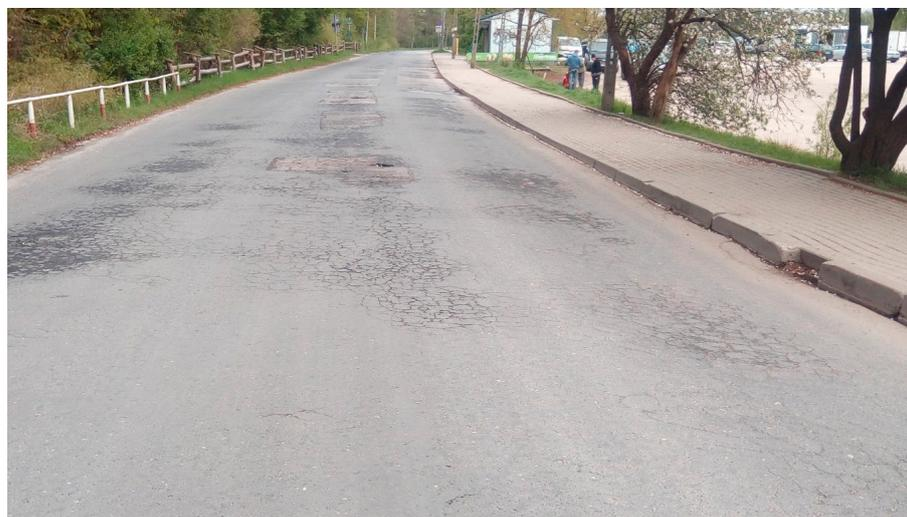
**Figure 1.** Deformed ground under road surface (Piechowicz, K. Bumps on the Road [Photograph]; 2024).
