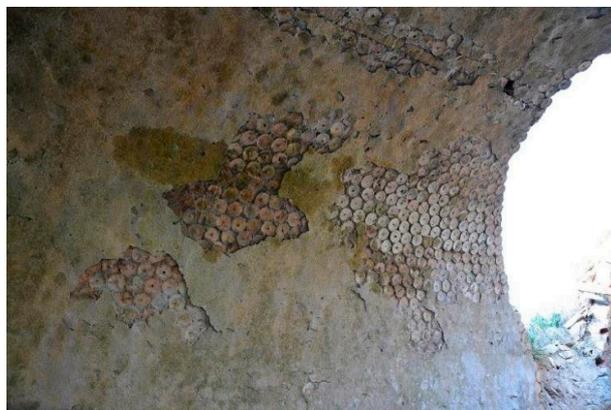
**Figure 8.** *Jazzo "Del Demonio"* (Italy)—lightweight vault made with hollow cylinders.
