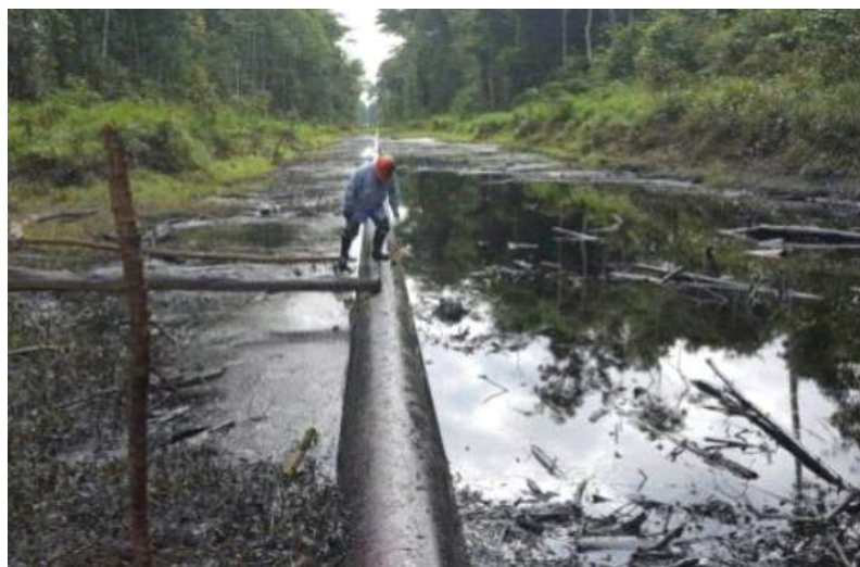
Figure 9. Section of an image of a lane built in the vicinity of the Marañón River in order to support an oil pipeline. The pipeline, in the middle-bottom of the image, suffered a severe disruption on 22 August 2016. As a consequence, the lane and the Marañón River received high quantity of crude oil causing an environmental disaster ( 4^{\circ}48'45.6''\text{S} 75^{\circ}23'56.8''\text{W} ) [87]. The image shows the crude oil around the pipeline. Source: http://geoportal.regionloreto.gob.pe/mapa-de-derrame-de-petroleo-en-el-tramo-i-del-oleoducto-norperuano/ (accessed on 9 July 2018).
