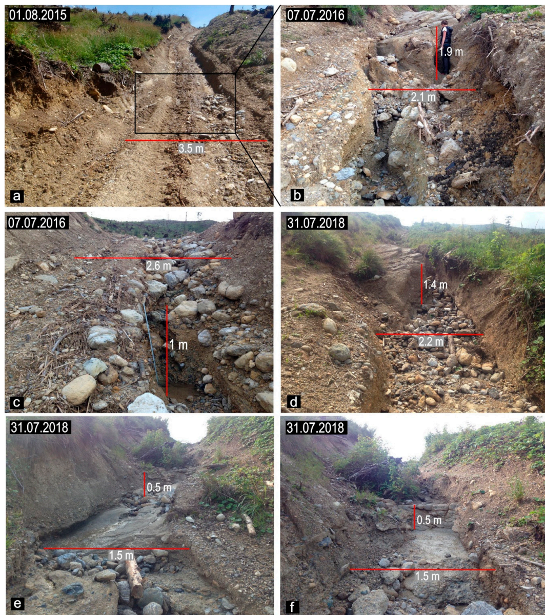
Figure 2. Changes on the surface of the studied road, explanations: the road in use in the first year after its construction (a); deep incisions formed after heavy rainfall, which contributed to exclusion the road from usage (b,c); strong relief transformations on the road two years after exclusion the road from usage (d–f).
