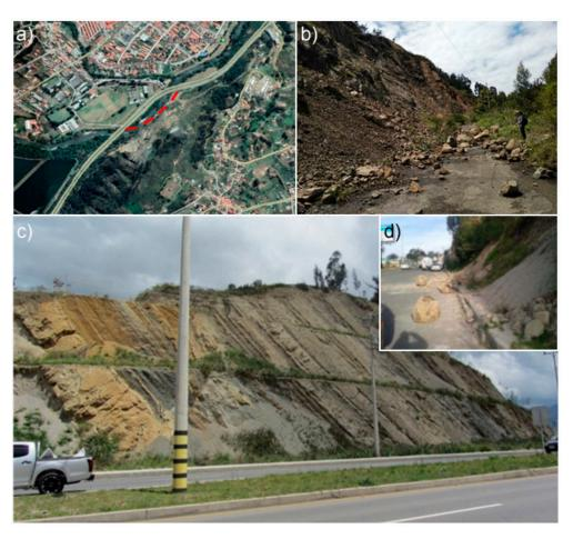
**Figure 2.** The functionality of the Pan-American Highway is often interrupted by rockfalls. (**a**) Deviation of the original road axis (red dotted line) caused by rockfall events; (**b**) landslide deposits have almost completely invaded the highway; (**c**) overdip cataclinal slope: the stratification is slope-oriented; (**d**) boulders detached from the slopes block the lane.
