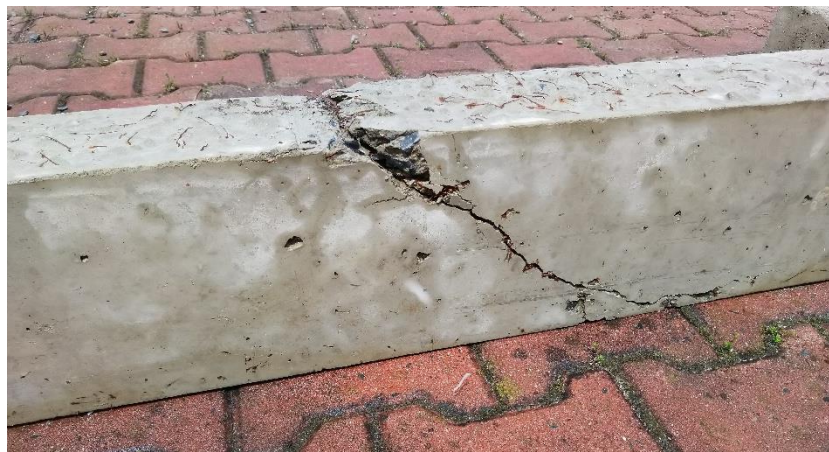
Figure 21. Details of a shear crack.
