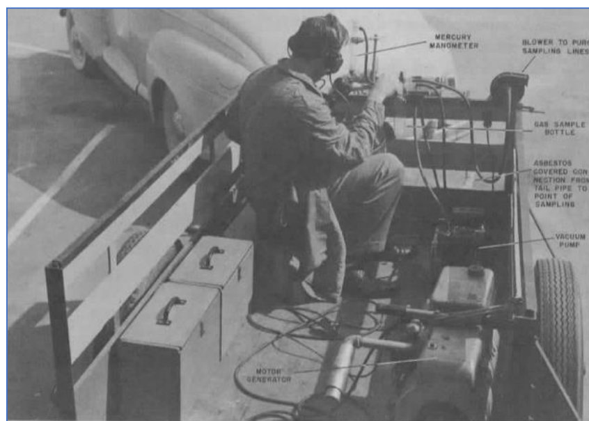
Figure 10. SIR exhaust sampling trailer attached to test vehicle [31].
