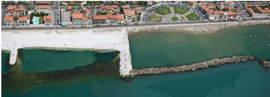
**Figure 14.** Marina di Pisa: on the right the old defence system with revetments and detached breakwater and on the left the new one with gravel beaches and submerged breakwaters (Photo Provincia di Livorno).
