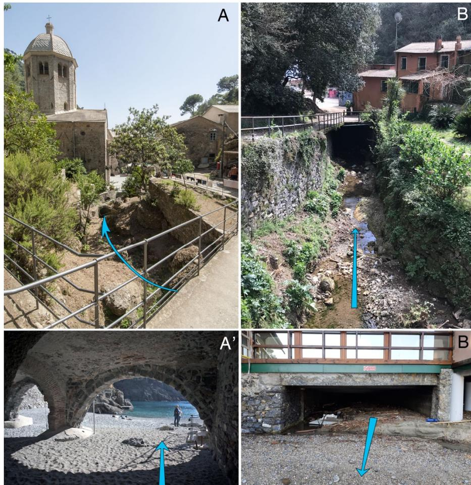
**Figure 9.** Culvert inlets (A,B) and outlets (A',B') at the stream mouth in catchment n. 2 for A–A' and catchment n. 5 for B–B'.
