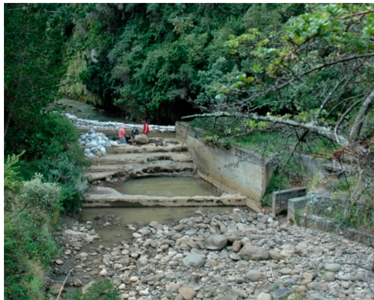
Figure 7. The water intake for the El Calvario canal in the community of La Chimba in the dry season and the riverbed that runs out of water for the other community concessions.
