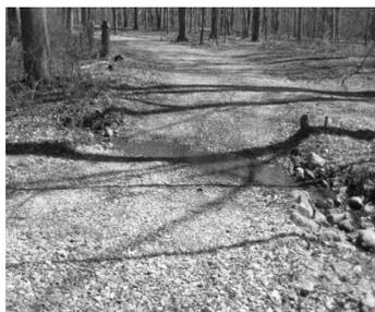
**Figure 3.** Ford crossing with BMP+ treatment, including rocky running surface and Geo-Web in the channel.
