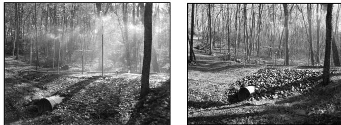
**Figure 2.** **Left:** Culvert after installation and during BMP– rainfall simulation; **Right:** Culvert prior to BMP+ rainfall simulation with rocky running surface and fill slopes and seed and mulch on bare soil.
