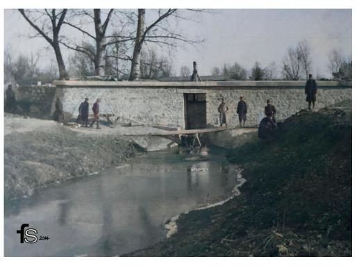
**Figure 4.** View of the damming wall of the *Wilga-Schleuße* fortress weir, seen from the side of the inundation area. Archival photograph from 1915. From the author's collection.
