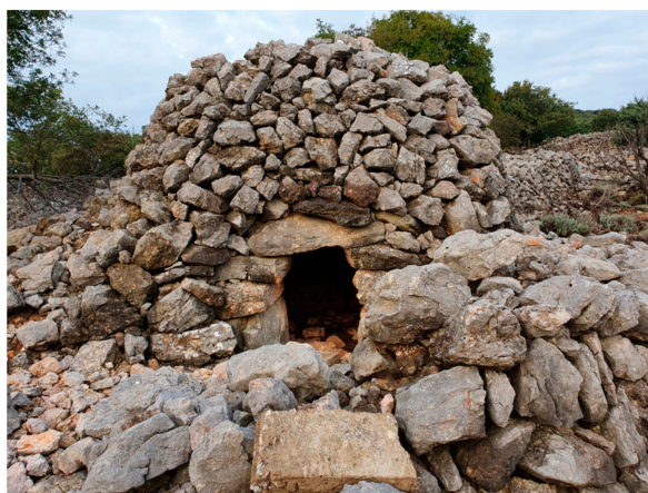
Figure 24. Dry stone shelters with round plans and stone roofing are considerably less frequent and less known on the islands of Cres and Lošinj in comparison to the rest of the Croatian coast (Tanja Kremenić, 2020).
