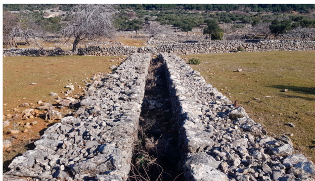
Figure 21. The dry stone channels serve to direct the water from the heavy rainfalls and flooding (Tanja Kremenić, 2020).
