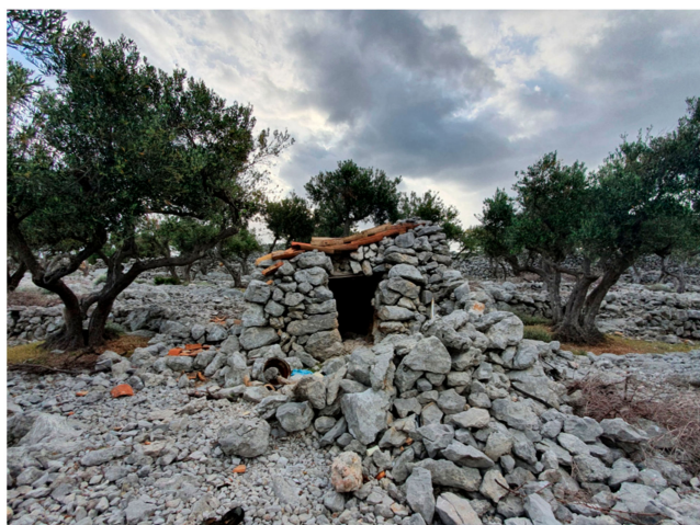
Figure 23. The typical dry stone wall shelter, with a maintained single pitch roof made from tiles, is in the Cres olive grove (Tanja Kremenić, 2020).
