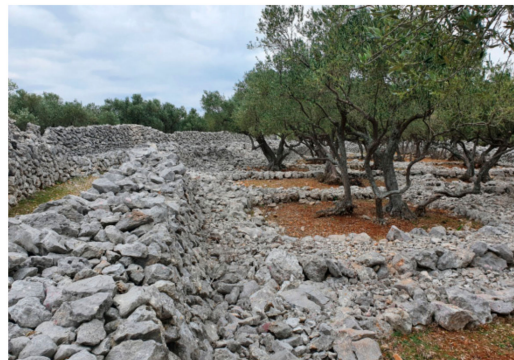
Figure 18. From left to right: a dry stone wall pathway, higher double wall ( gromača ), lower dry stone walls ( barbakan ) (Tanja Kremenčić, 2020).
