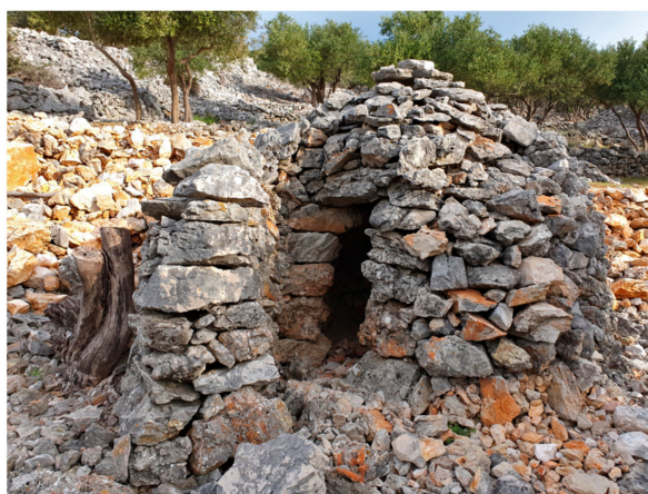
Figure 25. Besides being rare, dry stone shelters with round plans and stone roofing differ among themselves (Tanja Kremenić, 2020).
