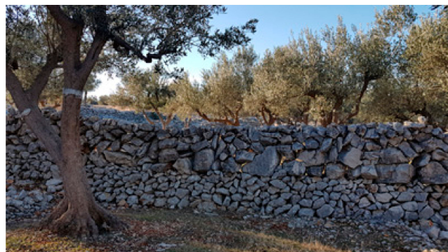
Figure 19. Island of Cres specificity—a dry stone wall of combined construction, composed of both a double and single dry stone wall (Tanja Kremenčić, 2020).
