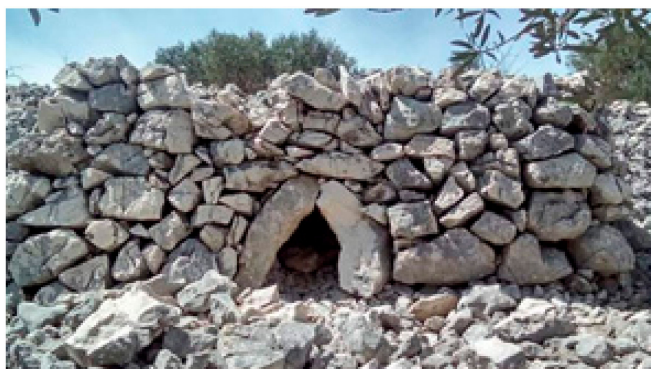
Figure 26. A stone pile with a dry stone wall on top (Goran Andlar, 2016).
