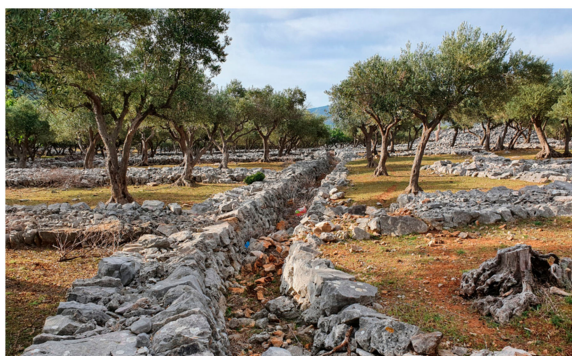
Figure 20. The drainage system within the Cres olive grove consists of dry stone channels which gather the water from the terraces, thus avoiding the rainfall to damage the yield (Tanja Kremenić, 2020).
