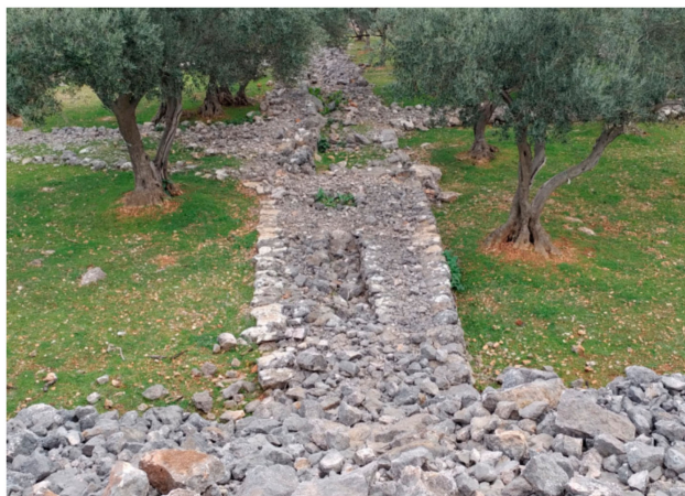
Figure 28. Dry stone details: a hole intended for lowering the donkey's height on which the bag with olives or grapes was placed (Franko Fučić, 2020).
