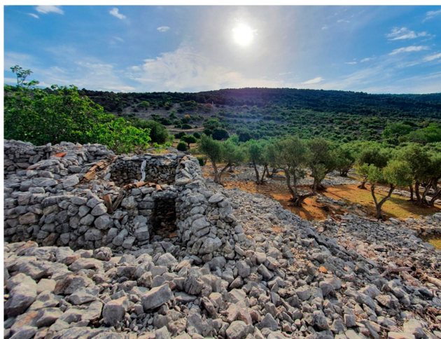
Figure 22. Dry stone wall shelters are for the most part rectangular and constructed on dry stone piles (Tanja Kremenić, 2020).
