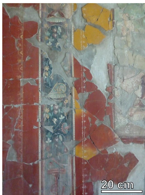
Figure 4. Detail of a portion of the east wall of the tablinum, with evident signs of temperature-induced chromatic alteration of the original yellow ochre.
