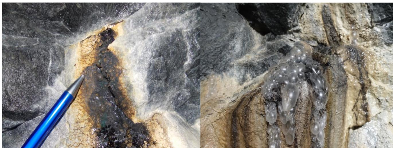
**Figure 2.** YBS with gas bubbles on the tunnel wall beneath the opening of a water-bearing fracture.
