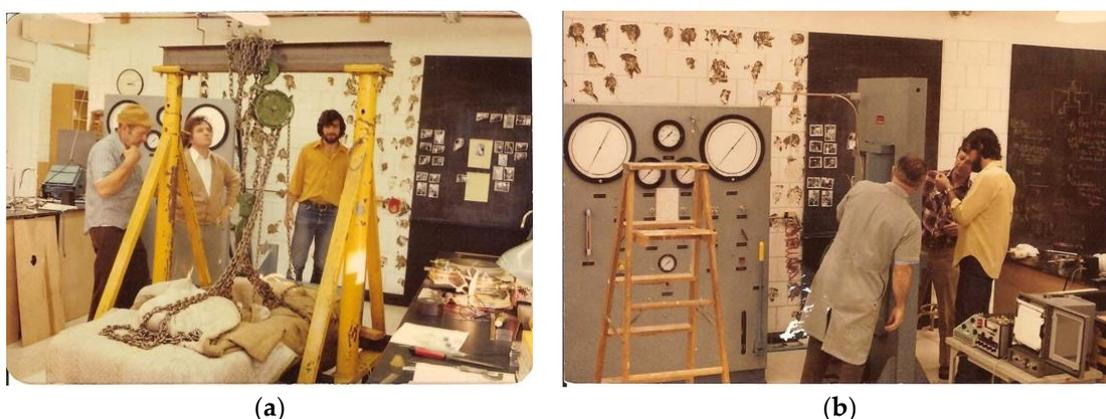
**Figure 1.** Installation of Harwood 500-ton press and girdle-anvil apparatus in 1977. (a) Bob and technician Tony Vidmar contemplating how to bring the press to upright position; (b) Al Catalano (machinist extraordinaire) and Alan Major from ANU with Tony Vidmar checking hydraulic connections to press.
