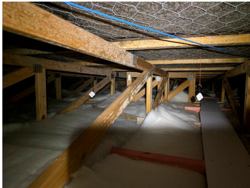
Figure 3. Roof space of the case study residential dwelling. Extensive mould growth is visible on the roofing underlay and the timber structure. Two hygrothermal sensors have been mounted in mid-air.
