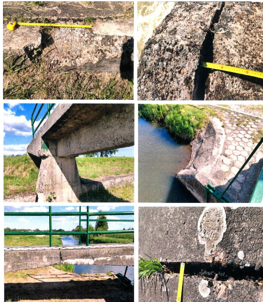
Figure 4. Technical condition of the Oświęcim Weir before renovation [30].
