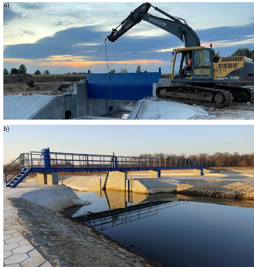
Figure 5. Remodelling (a) and functioning (b) of the Oświęcim Weir (source: State Water Holding Polish Waters).
