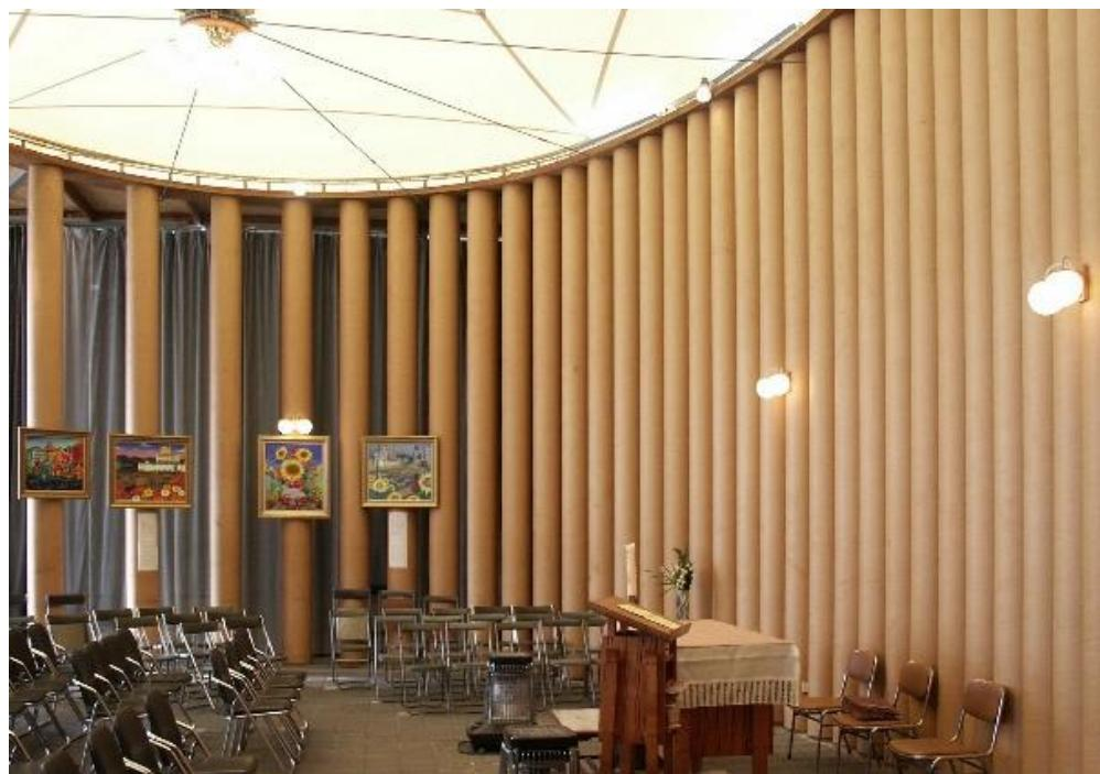
**Figure 5.** Use of cardboard as tube in construction (Takatori Catholic Church [64]).
