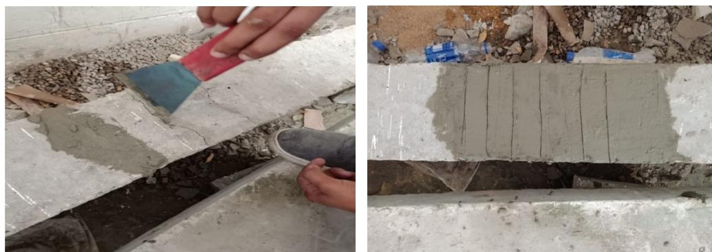
**Figure 7.** Application of Crack-Healing Solution with Cement Slurry on Beam “TCHS-3”.
