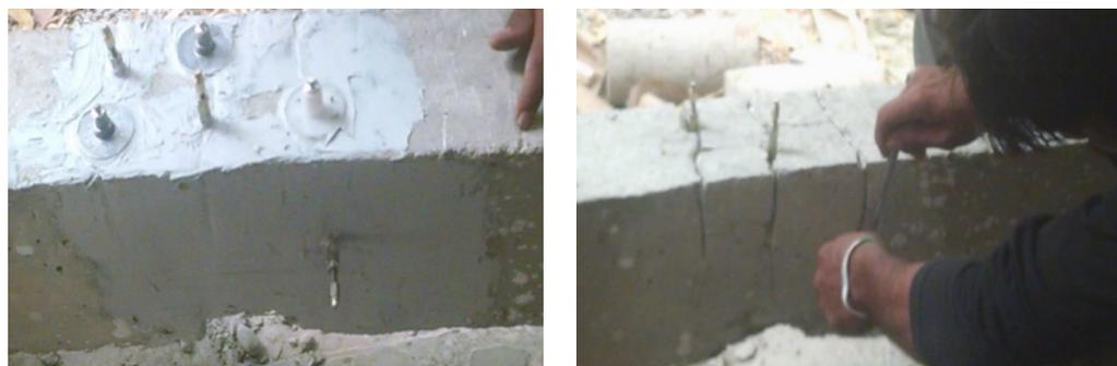
Figure 8. BASF epoxy resin application on Beam “TEIM”.
