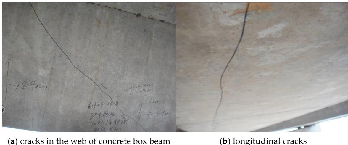
**Figure 4.** Typical cracks in the concrete box beams.
